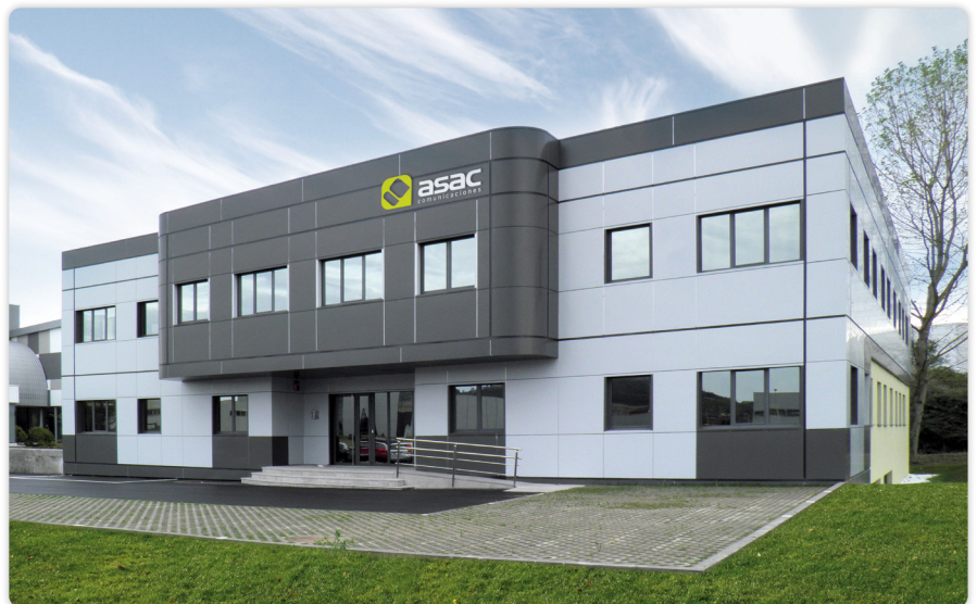
One of ASAC's buildings in Asturias where a Data Center is located.
